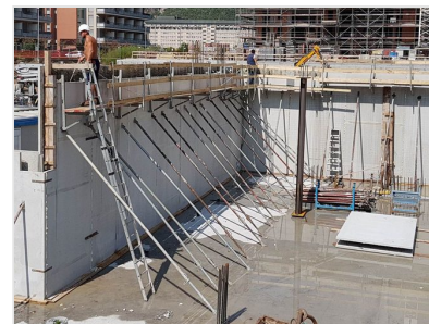
SOLAI E CASSEFORME IN OPERA
